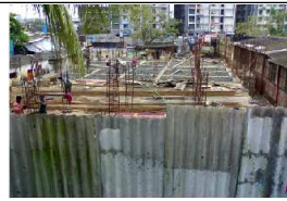
The ongoing construction at its plinth
